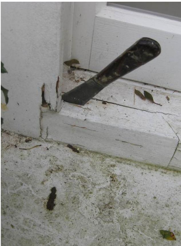
**Figure 5:** A sharp instrument is essential for investigating the extent of decay in a window. In this case, rot has occurred following the use of poor quality timber for a past repair. Photo: Joseph Bispham
